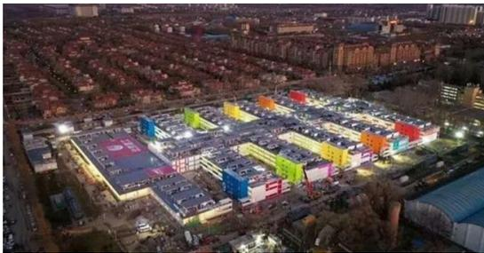
Fire-God Mountain, hospital: it is characterized by modular standard design, factory assembly line production, packaging and folding for transportation, and on-site modular assembly, which ensures the demand for short-term rapid construction.
