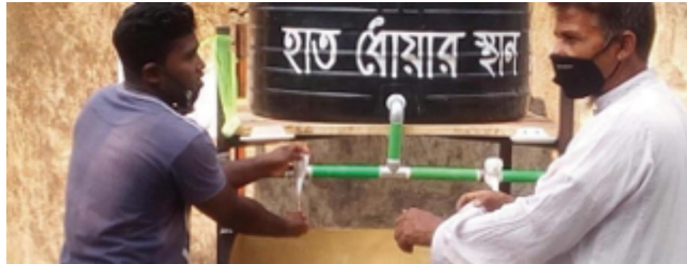
BANGLADESH | Faridpur Handwashing station installation in Ward no. 9
