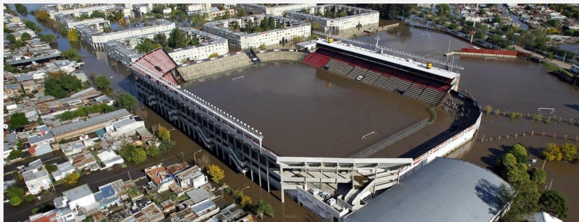
FIGURE 5 Flooding in Santa Fe in 2003
